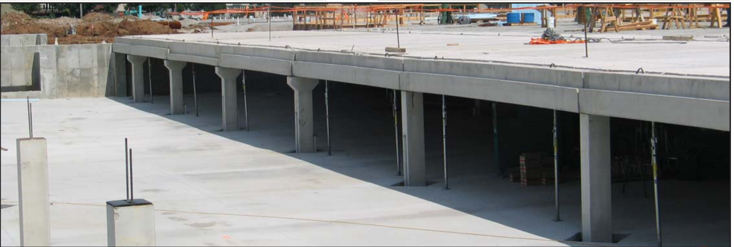
Pictured here are beams and columns supporting hollow core plank for the underground parking garage.
