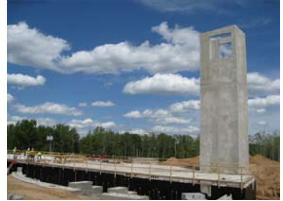
The Bell Tower stands almost 80' high
