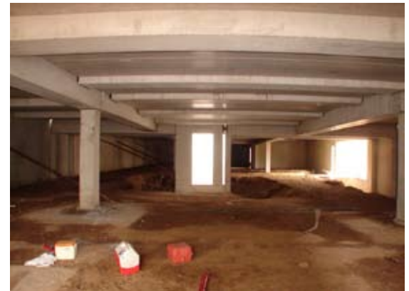
Precast transfer beams allowed the elimination of various columns
