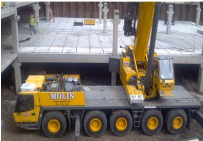
Molin's 120-ton crane was a perfect fit for erecting this project.
