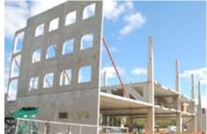
Pictured here are various Columns, Trusses, Hollow Core, Beams, and Walls that made up this complex job.
