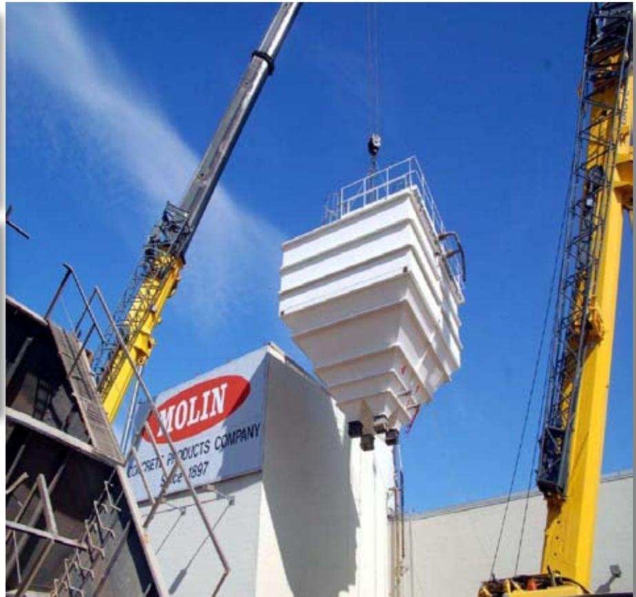
***The new aggregate bins were constructed over a six week period and have 400-ton capacity.***
