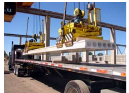
Hollow Core being loaded in one of our gantry bays
