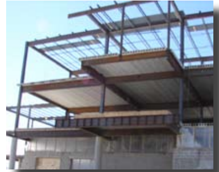
Hollow Core decking installs quickly in any weather condition
