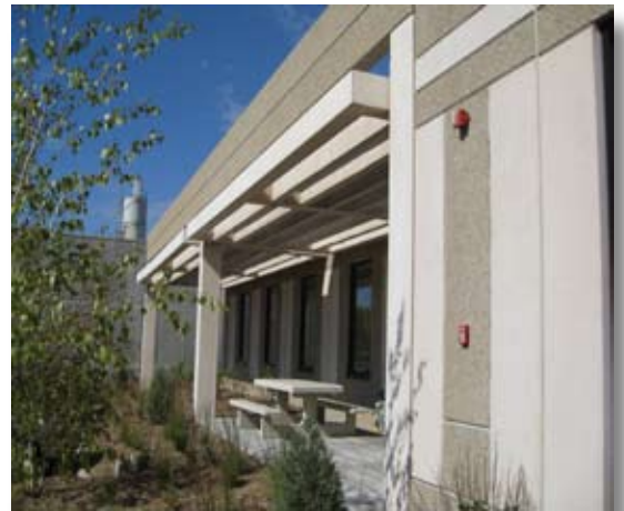
Molin Concrete custom-built this precast concrete sunshade to eliminate heat gain.
