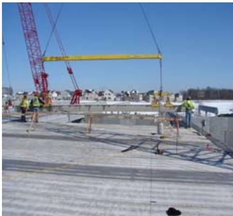
An integral part of the hollow core plank design was the FEMA F5 Tornado Design that the project specified. The design requires keyway bars, additional weld plate connections, and a detailed shear wall to hollow core plank connection.
