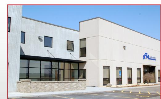
**DESIGN:** Molin successfully designed a three-sided expansion to an existing precast building at F & M Plastics. The panels are load bearing insulated sandwich panels with a rake finish. The design process included early collaboration with the design architect to create a panel layout that was both practical, functional and optimized for efficiency. Our wall panels allow for easy building expansion, thus minimizing future construction costs.
