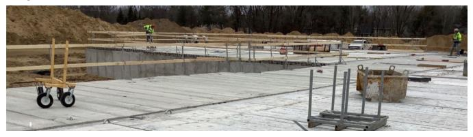
The guardrails we developed use 11-gauge steel stanchions (the vertical part of the guardrails) to support the weight of our workers and equipment. Foremen, bricklayers, and the rest of our installation team use them in the field. Workers can easily anchor our guardrails into the precast concrete because of the design. As workers move, so do the guardrails to keep the finished edge inaccessible. They are truly an innovation in precast workplace safety.
