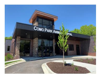
A total precast concrete structure increases energy efficiency through thermal mass, lowers maintenance, and simplifies the construction staging to accommodate tight site logistics.
